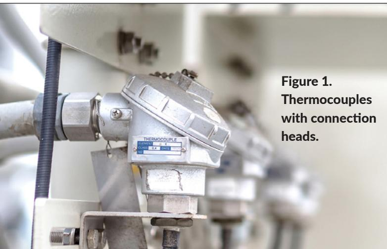
Figure 1. Thermocouples with connection heads.
