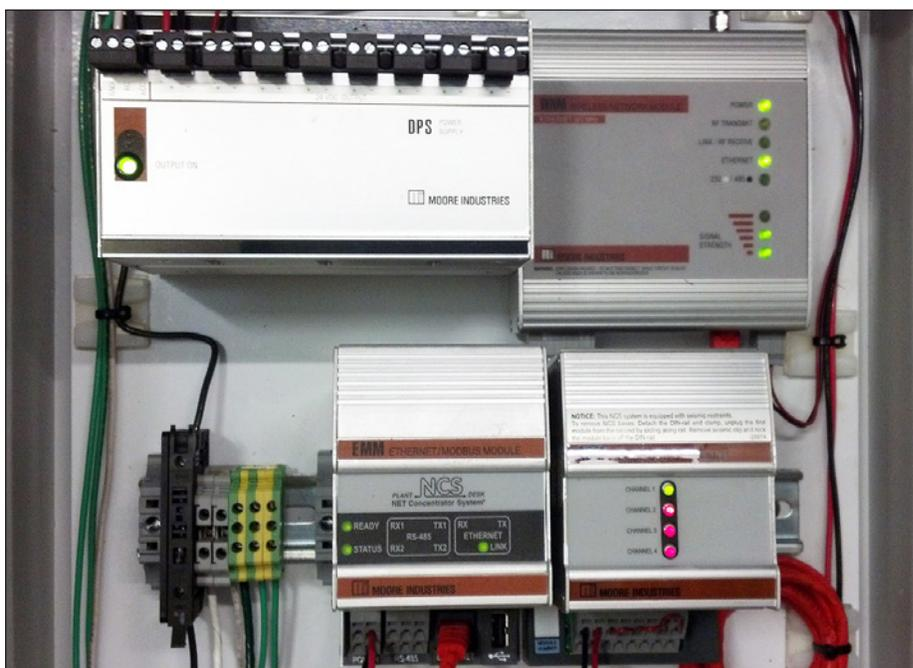
**Figure 4.** The wireless receiving panel installed at the boiler room of the pulp and paper mill. An Ethernet/MODBUS interface module (EMM) of the NCS serves as a MODBUS master to retrieve HART data from the HCS at the pond site.
