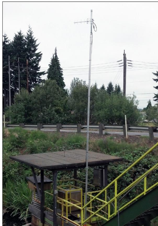
**Figure 3.** The Yagi-directional antenna was used at the pond site to transmit level signals from the HART level transmitter to the boiler room.
